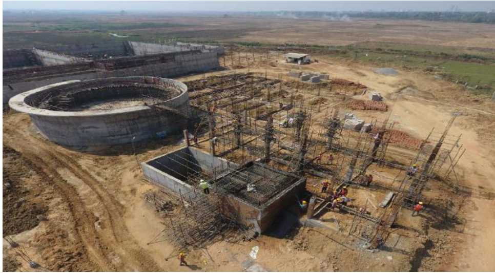
Fig. 10 Present Progress of construction of STP at Kochilaput (Sewerage District-III)
