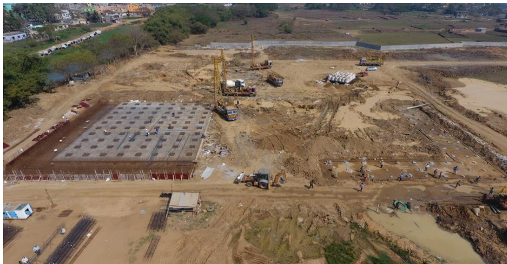
Fig. 8 Present Progress of construction of STP at Meherpalli (Sewerage District-I)
