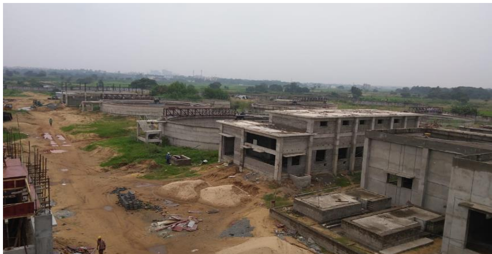
Fig. 12 Present Progress of construction of STP at Rokhat (Sewerage District-VI)
