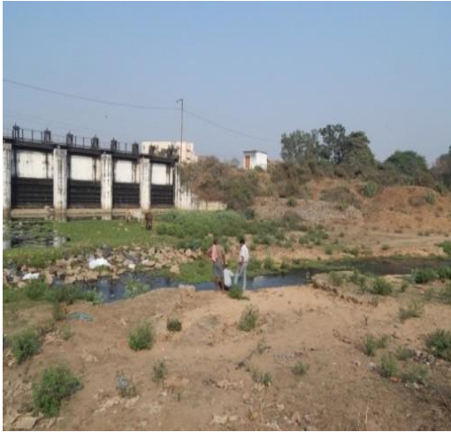
Fig. 3 Wastewater discharge to Kathajodi river near ABIT
