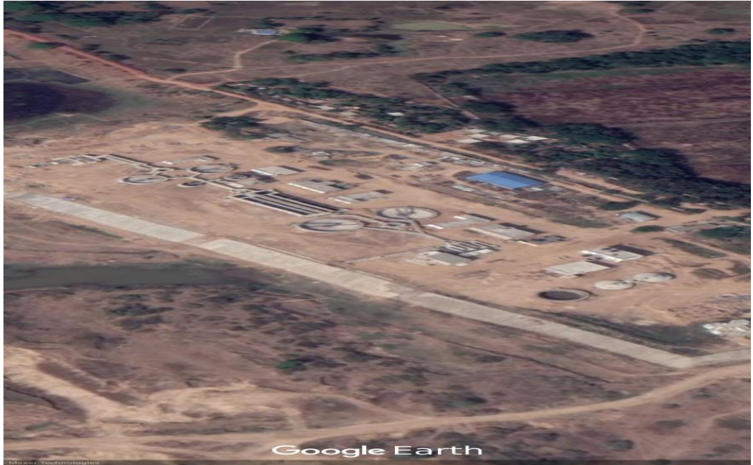
Fig. 10 Construction of 16 MLD STP at Mattagajpur
