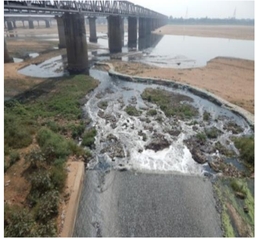
Fig. 4 Wastewater discharge to Kathajodi river at Khan nagar
