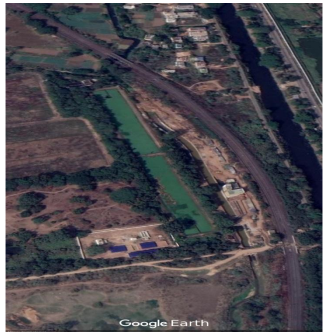
Fig. 11 33 MLD STP at Mattagajpur under renovation
