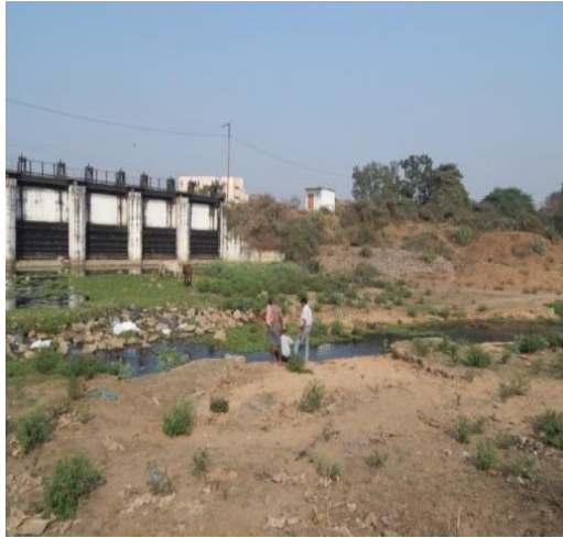
Fig. 3 Wastewater discharge to Kathajodi river near ABIT
