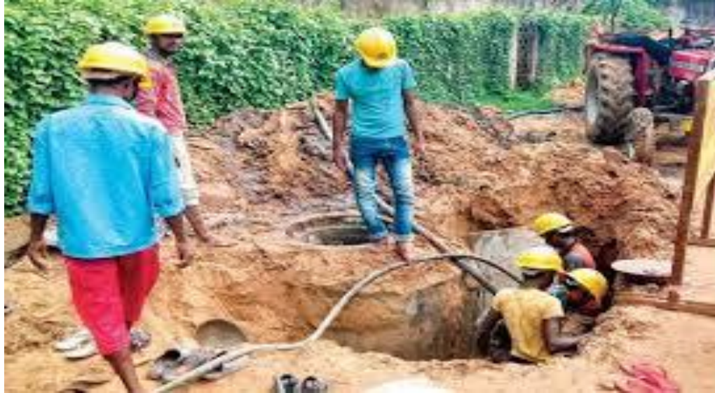
Fig. 12 Laying of sewerage line for household connection
